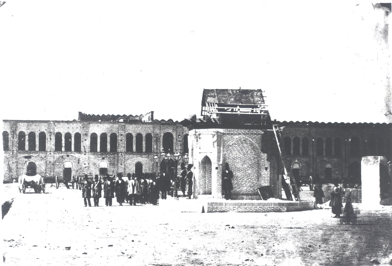
View of the building from the courtyard
